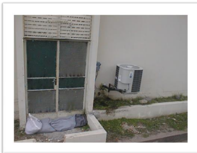
Fig. 11. Using sandbags in a flood prone area
